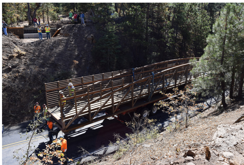
The finished bridge, ready to be crane-lifted and bolted into place.
