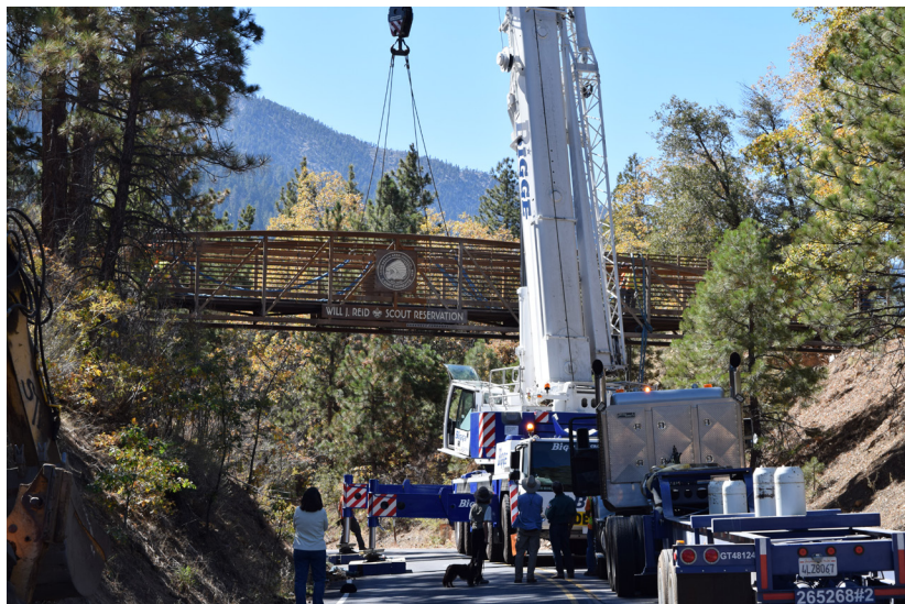
The crane positioning the bridge in place
