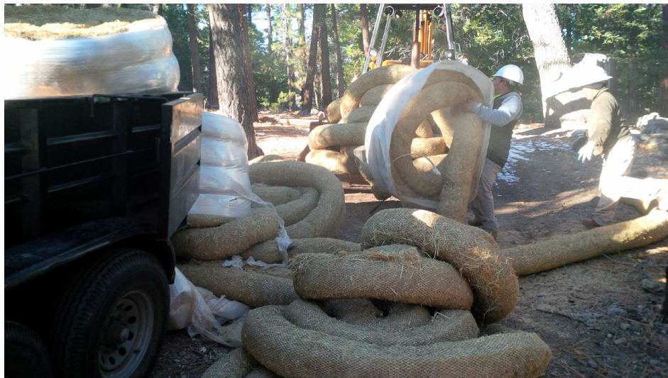
Erosion control efforts after the fire took miles of straw waddles
